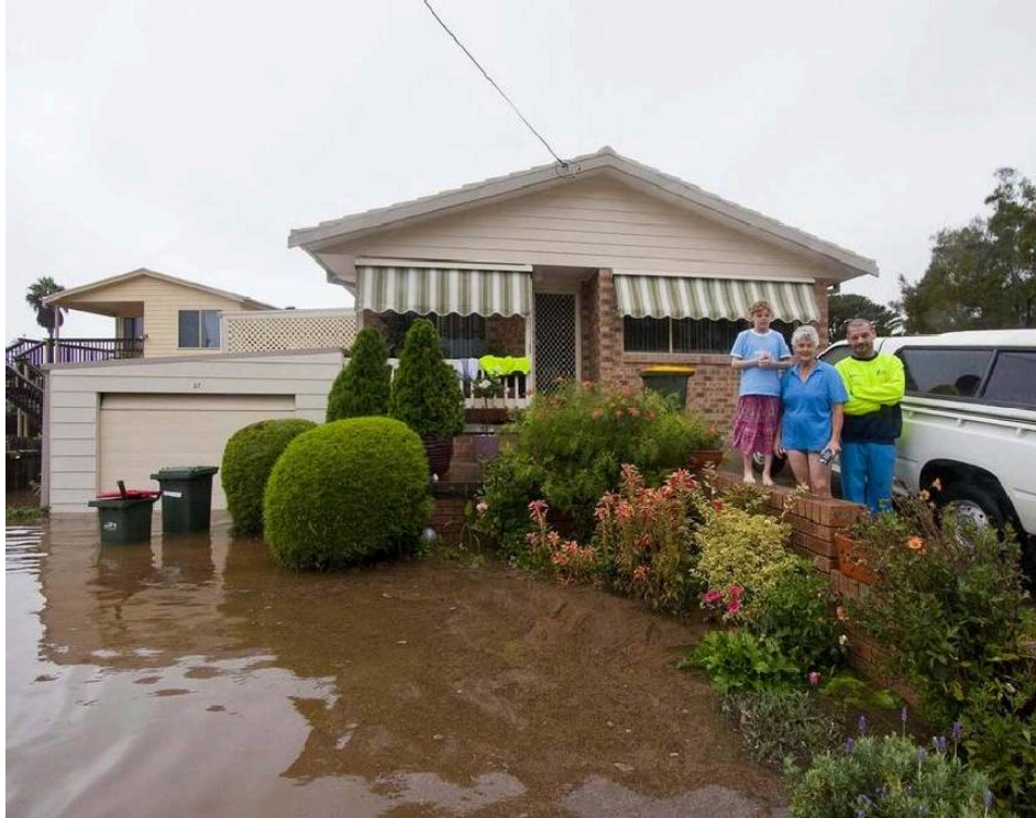
2010 Residential areas of Dalmeny already affected by flooding, adjacent to the proposed development
